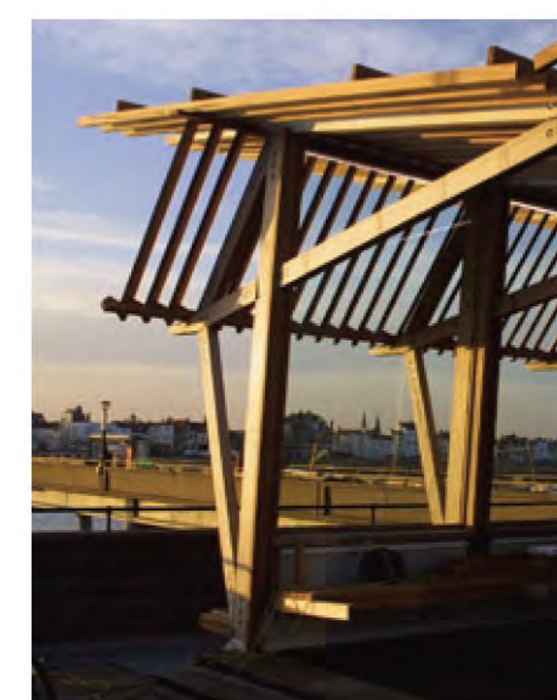
The Deal Cafe by Niall McLaughlin A wooden pavilion made from prefabricated frames of iroko hardwood which are greying nicely into similar tones as the concrete. It is designed to be transparent, allowing views through and around the building to the sea beyond.
