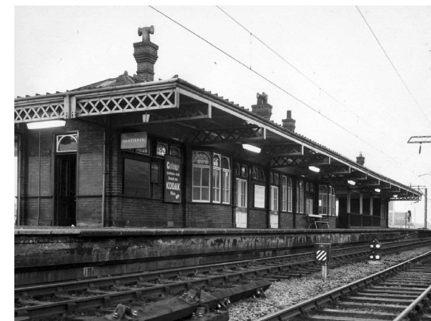
12. Dumbarton station platform mid-20th century
